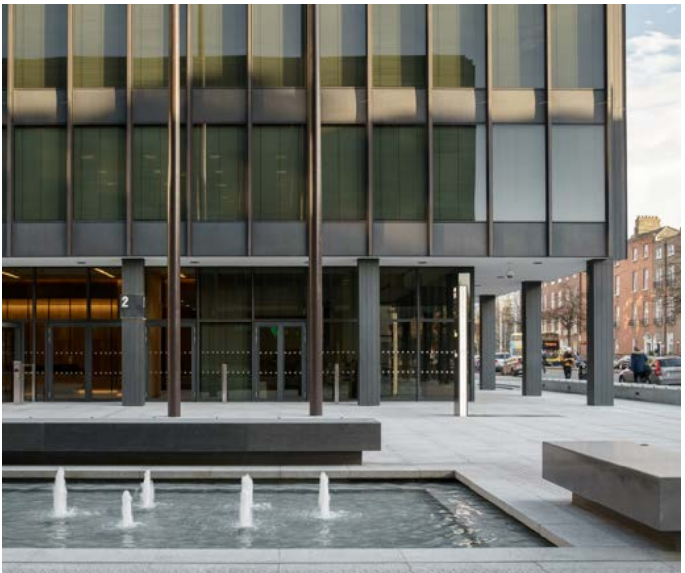
Renovated facade at Miesian Plaza
